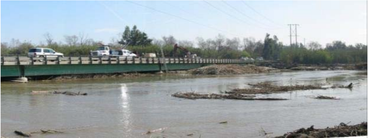
Figure 8 Image of Completed River Road Bridge (Before Construction)
