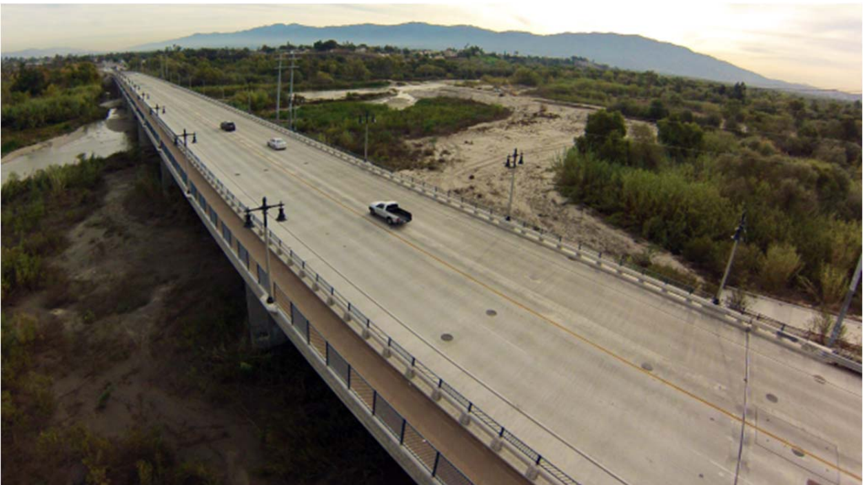
Figure 9 Image of Completed River Road Bridge (After Construction)
